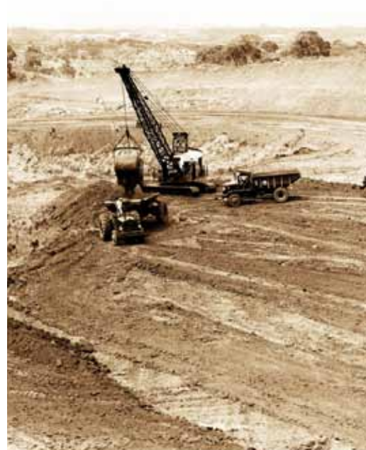
Third Locks Program - Dry Excavation at Gatun, Canal Zone.
